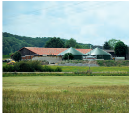
Biogasanlage in Großen-Buseck
